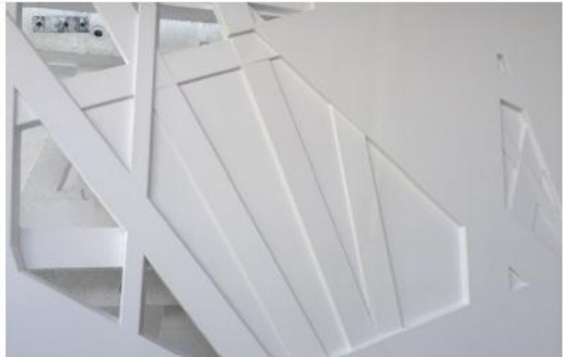
Figure 48. The final shape is realized by using biodynamic fiberglass reinforced concrete.
