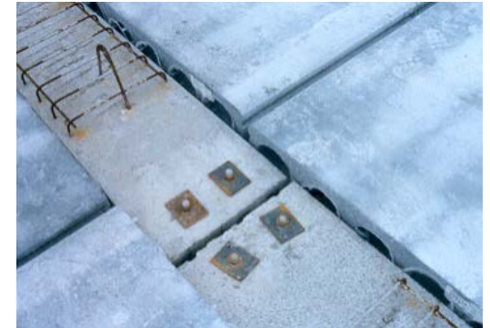
Floor beams to columns
