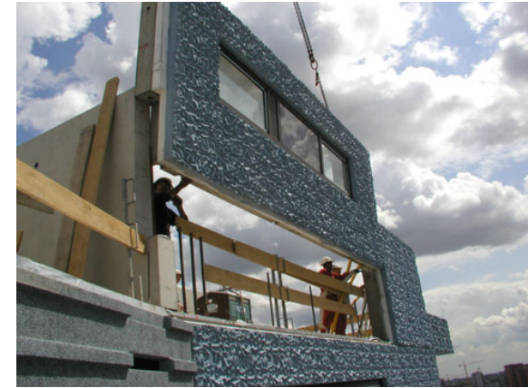
Storey high panels
