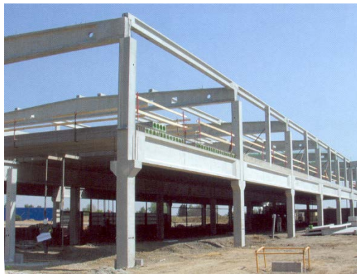
Portal frames with intermediate floor
