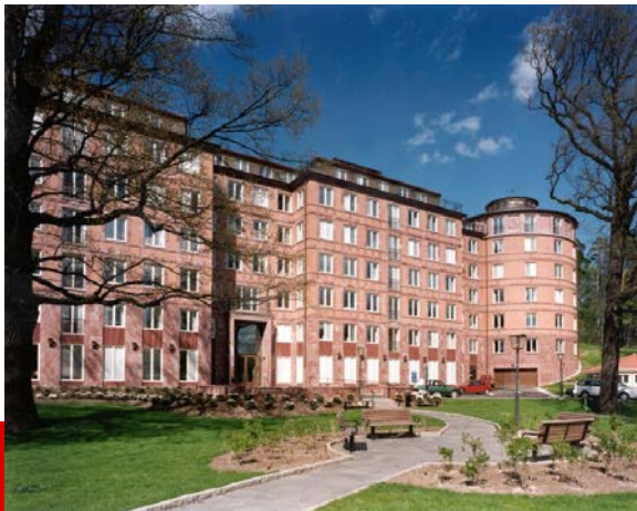
Façades in precast concrete
