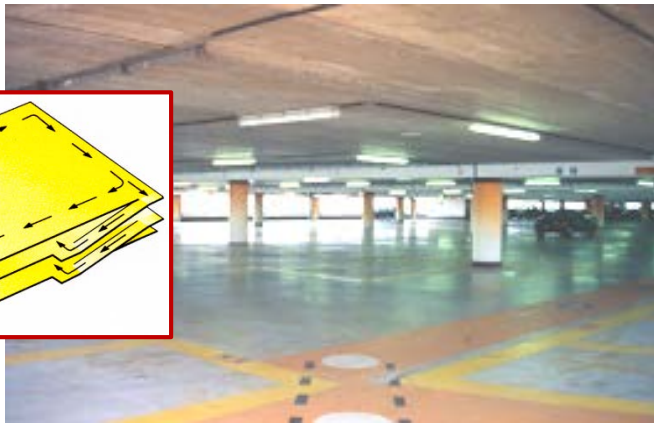
Flat parking deck
