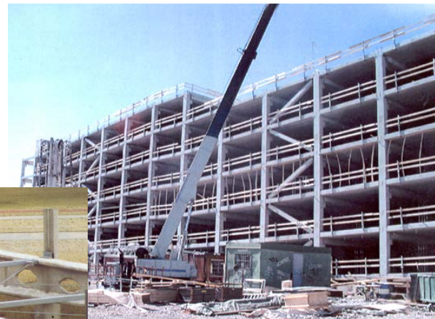
Steel diagonal cross bracing
