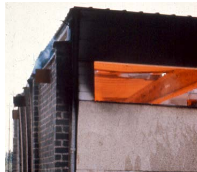
Failure test roof beam after repair
