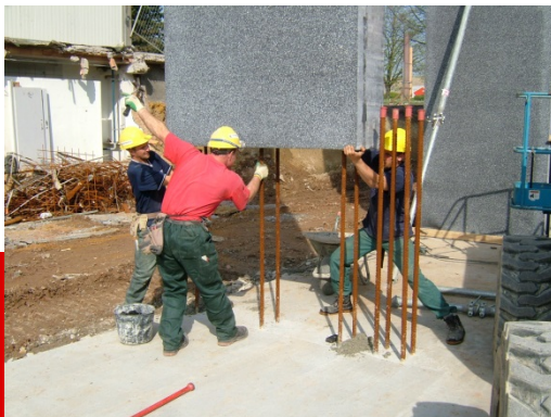
Projecting bars in grout holes
