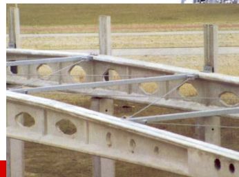
Steel diagonal cross bracing
