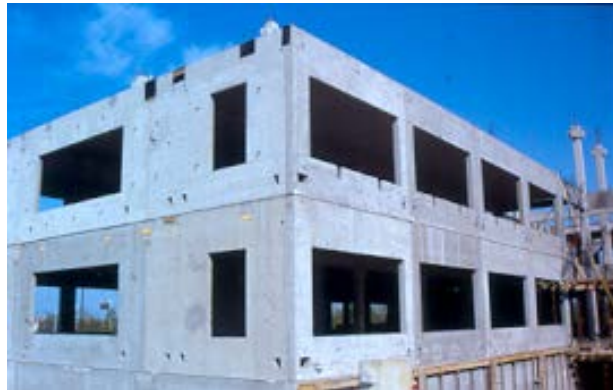
Stability through cross wall action
