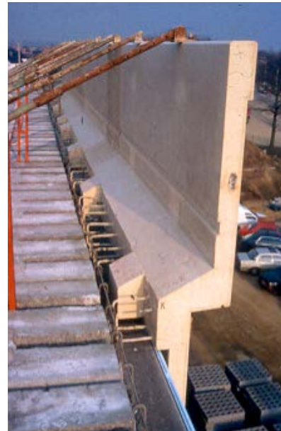
Projecting bars with in-situ concrete
