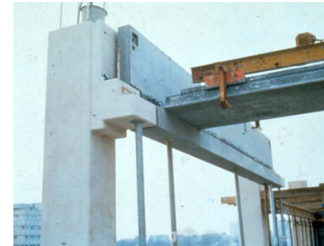
Spandrel beams
