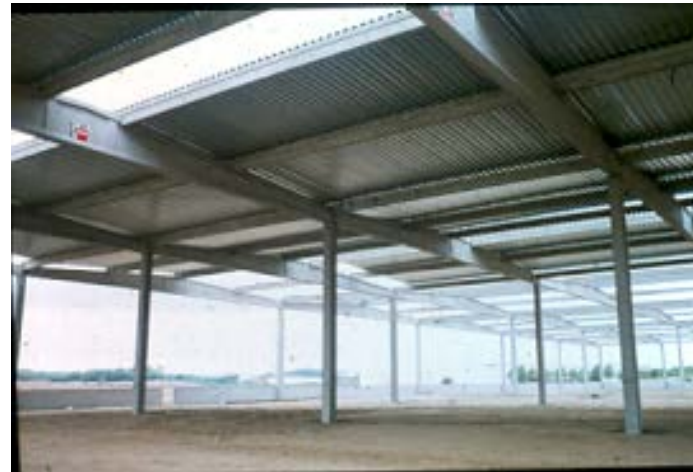
Portal frames with purlins
