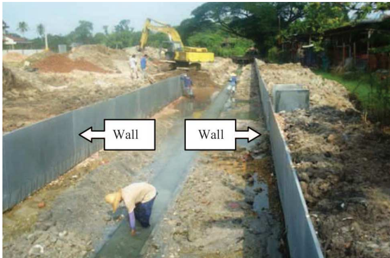
Construction of retaining wall for drain channel in Ipoh, Malaysia,
