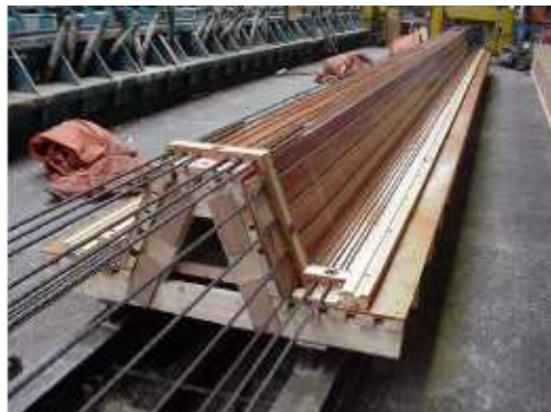
Fig. 10 Mould with strands for pile production
